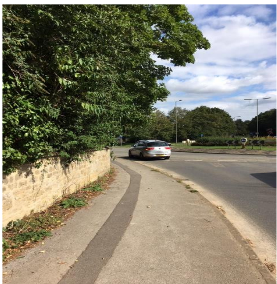
Driver's view of crossing point is obstructed by foliage and wall.
